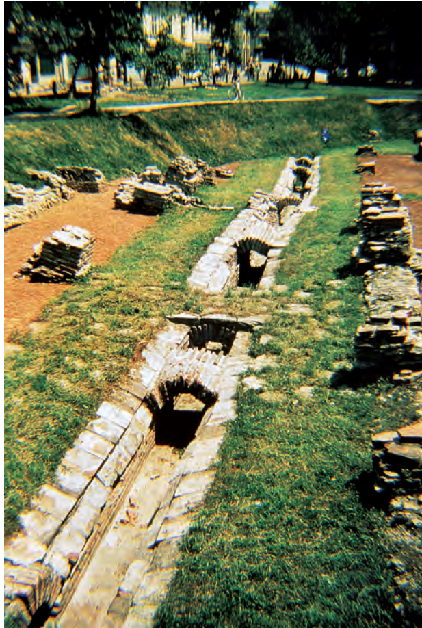
Fig. 8: The street canalization
